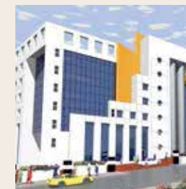
SILICON PLAZA PUNE
